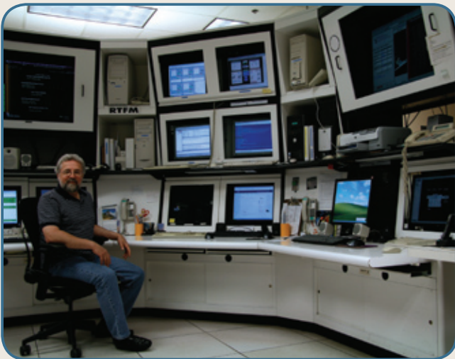
David Rohwer, Manager of Data Center Operations is keeping an eye on the university computer systems and equipment. Photo by Nile Mueller.
