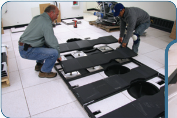
OIT staff carefully install ISO-Base™ platforms for new computer racks. Photo by Monique Musick.
