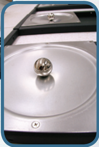
Heavy-duty ball bearings keep computer racks from tipping when the ground is shaking (likes weebles, they wobble, but they won't fall down). Photo by Monique Musick.
