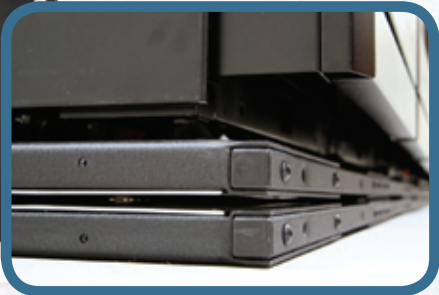
OIT staff carefully install ISO-Base™ platforms for new computer racks. Photo by Monique Musick.
